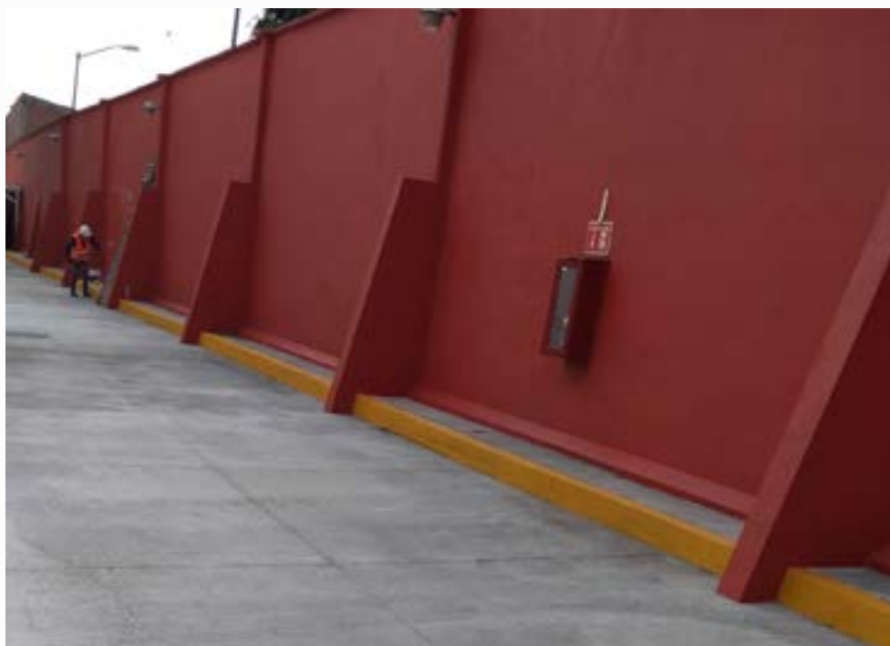
Barda perimetral reparada
